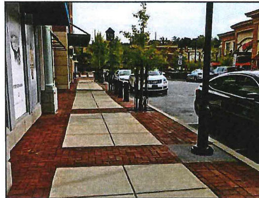
Sidewalks utilizing Unit Pavers
