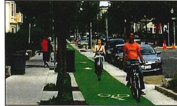
Bicycle Lane and Markings
