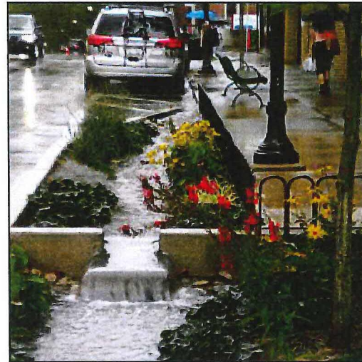
Bioswale along street providing Stormwater Management
