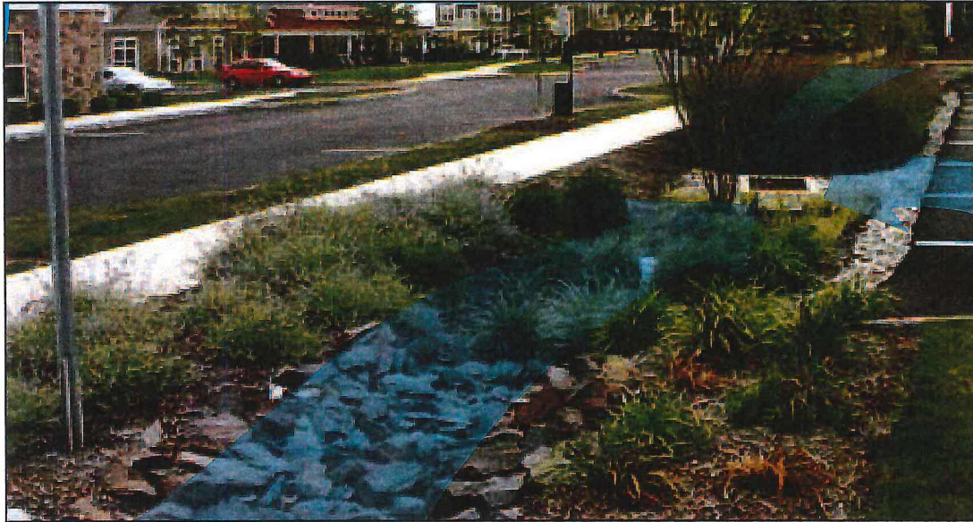
Bioswale in parking lot "cleansing" stormwater before infiltration
