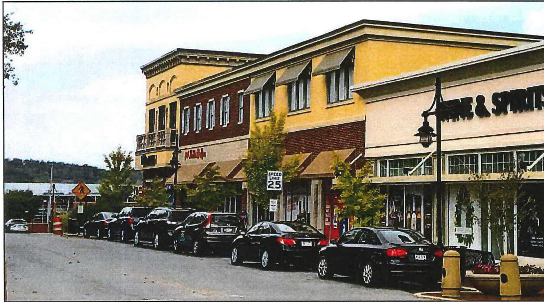
Buildings located at Build-To Line with on-street parking, and a parking lot in the rear
