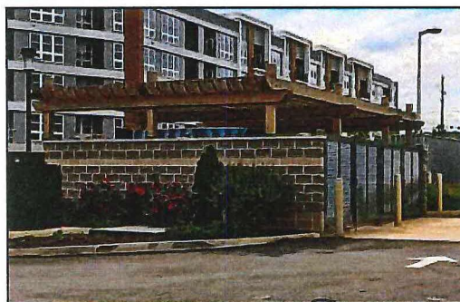
Dumpster screened inside enclosure
