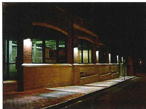
Wall Mounted Lights diffused in downward orientation
