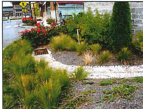
Stormwater infiltration system in parking area
