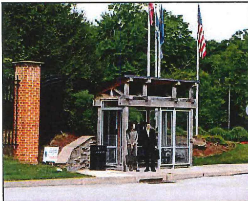
Bus Shelters in close proximity to businesses and multi-family dwellings
