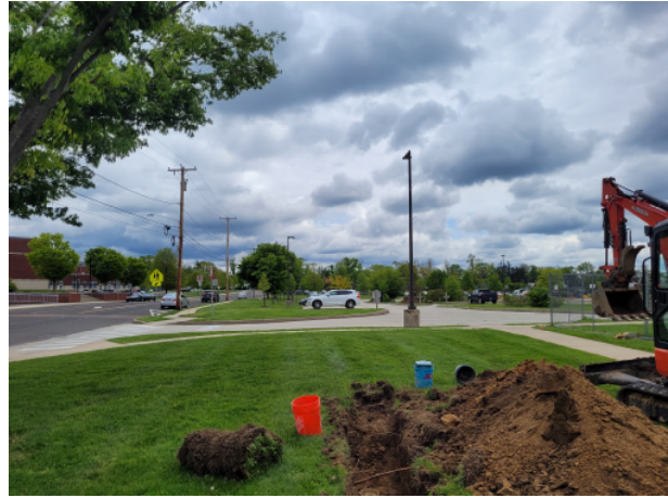
Photograph 4 – Looking Southeast from Test Pit Location TP-106
