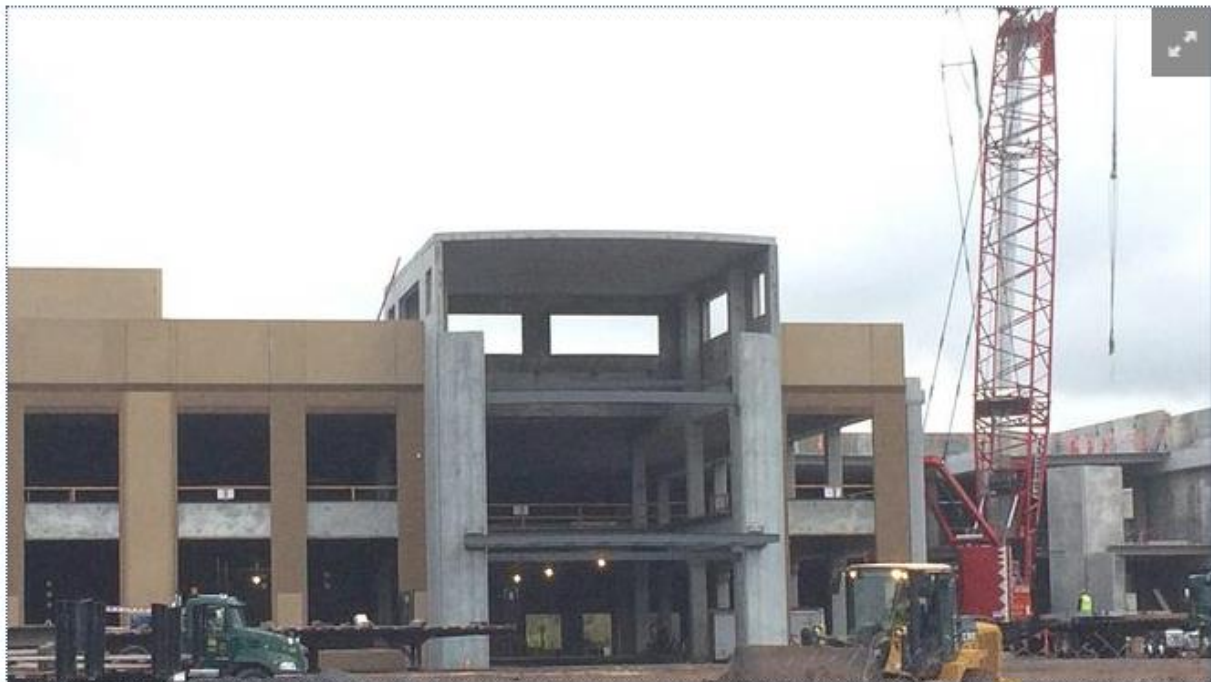
Lifetime Fitness under construction at Fort Washington Office Park.
