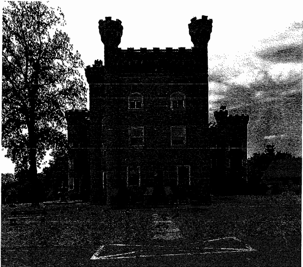
East Elevation: The building's three-story rear ell faces east with a two-bay elevation bracketed by slender blind corner turrets crowned by ornamental battlements. A single-leaf wood door is centered on the ground floor, accessed by a narrow stone stoop framed by thick sidewalls.
