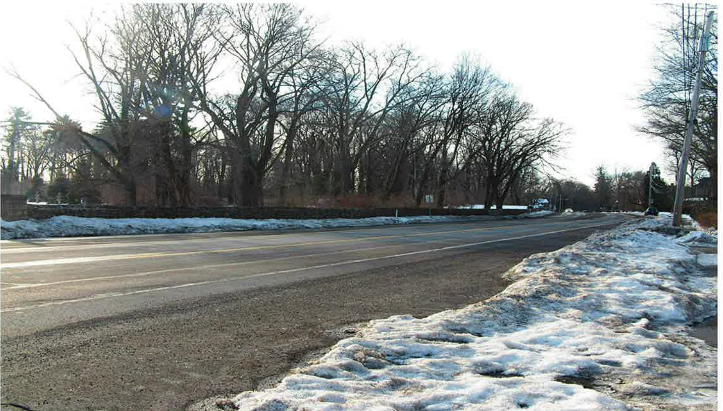
Wall along Bethlehem Pike looking southeast from Lindenwold Avenue
