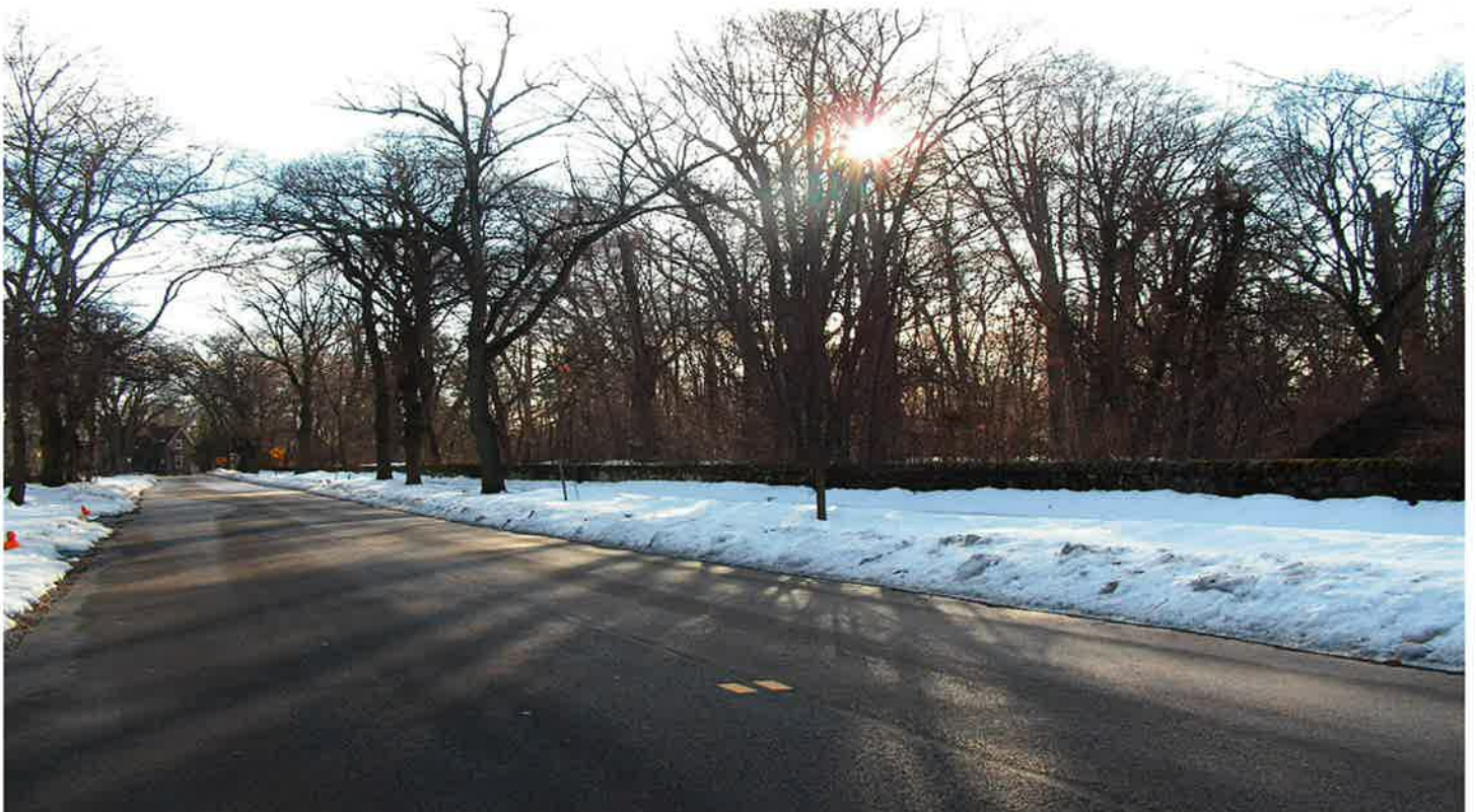
Wall along Lindenwold Terrace looking southeast
