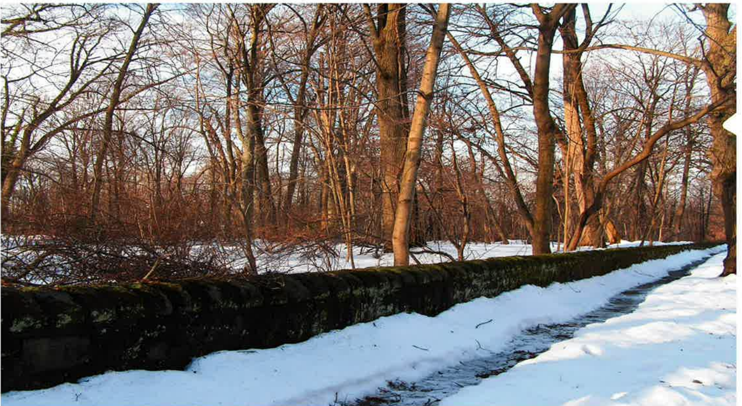
Wall along Lindenwold Terrace looking southwest
