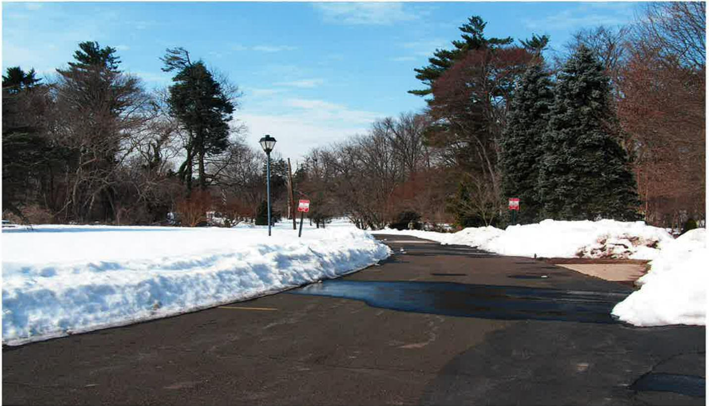
Main Driveway from Castle toward Bethlehem Pike and Lindenwold Terrace
