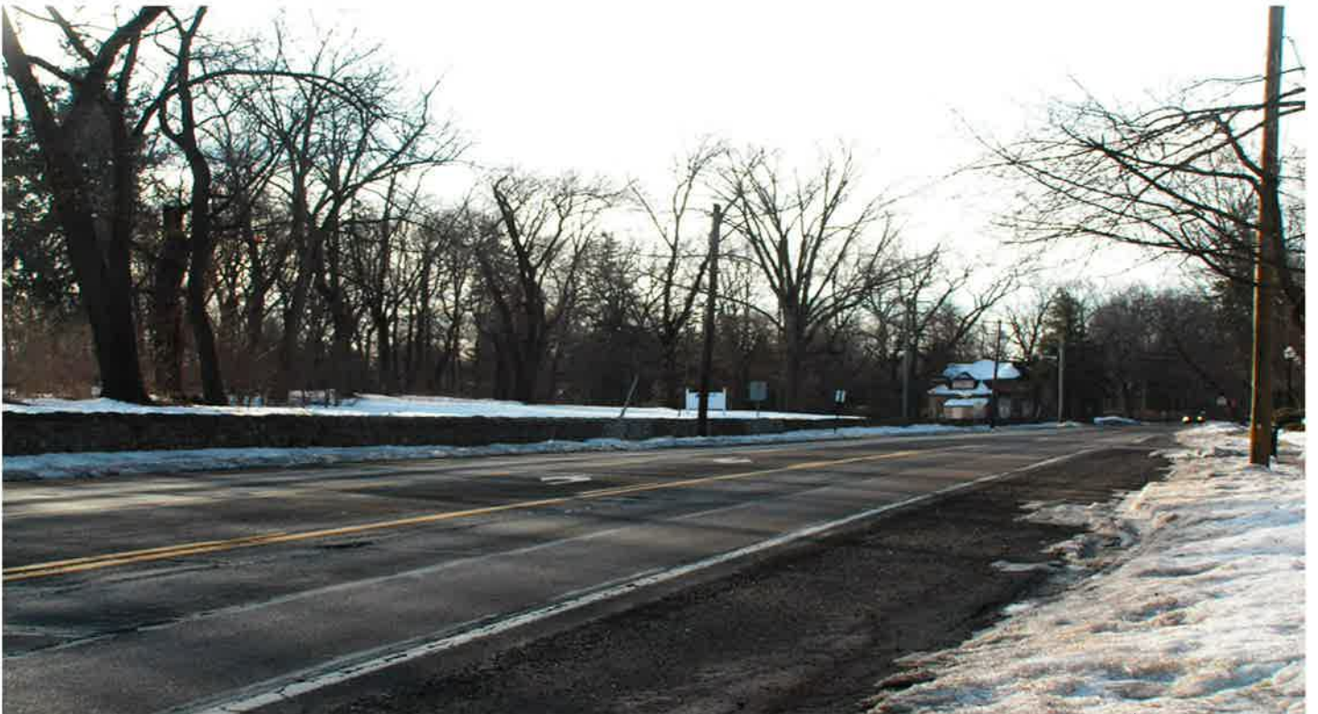
Wall along Bethlehem Pike looking southeast near Mattison Avenue
