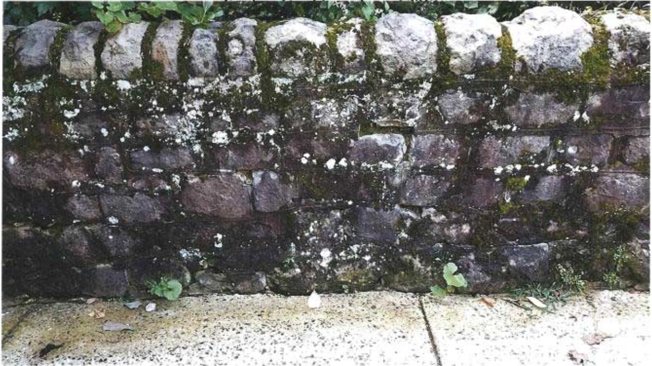
Lindenwold Terrace perimeter wall: A low fieldstone wall marks the perimeter of the property along Lindenwold Terrace. The wall generally features random ashlar and rubble coursing topped by semi-rounded capstones. It sits adjacent to a concrete sidewalk running parallel to Lindenwold Terrace.
