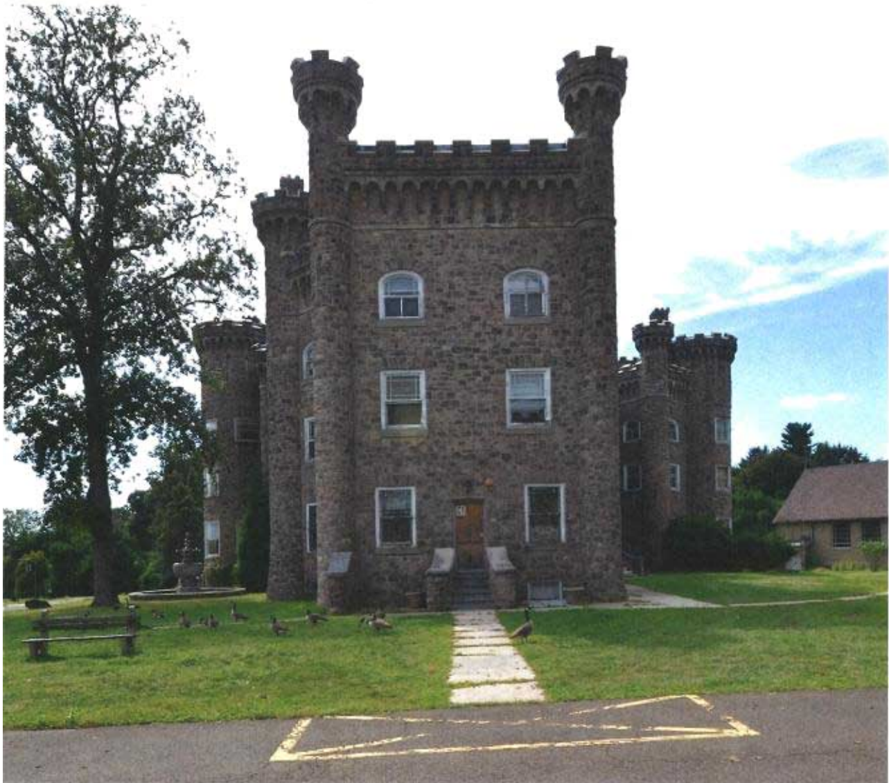
East Elevation: The building's three-story rear ell faces east with a two-bay elevation bracketed by slender blind corner turrets crowned by ornamental battlements. A single-leaf wood door is centered on the ground floor, accessed by a narrow stone stoop framed by thick sidewalls.
