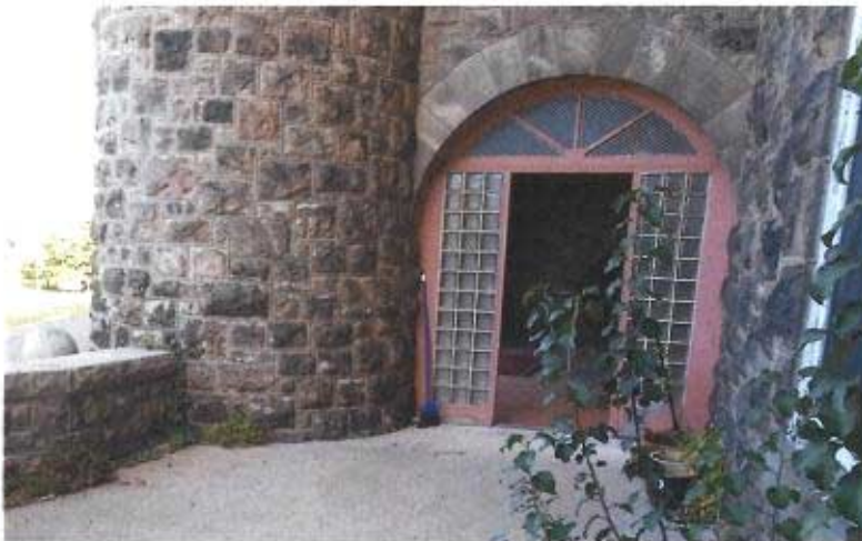
West Elevation Details: An arched doorway connects porch to a raised, open patio to its north. The doorway features a glazed fanlight transom and glass block sidelights in wood frames, but no central leaf. The patio features a concrete floor and a low stone-capped perimeter wall.
