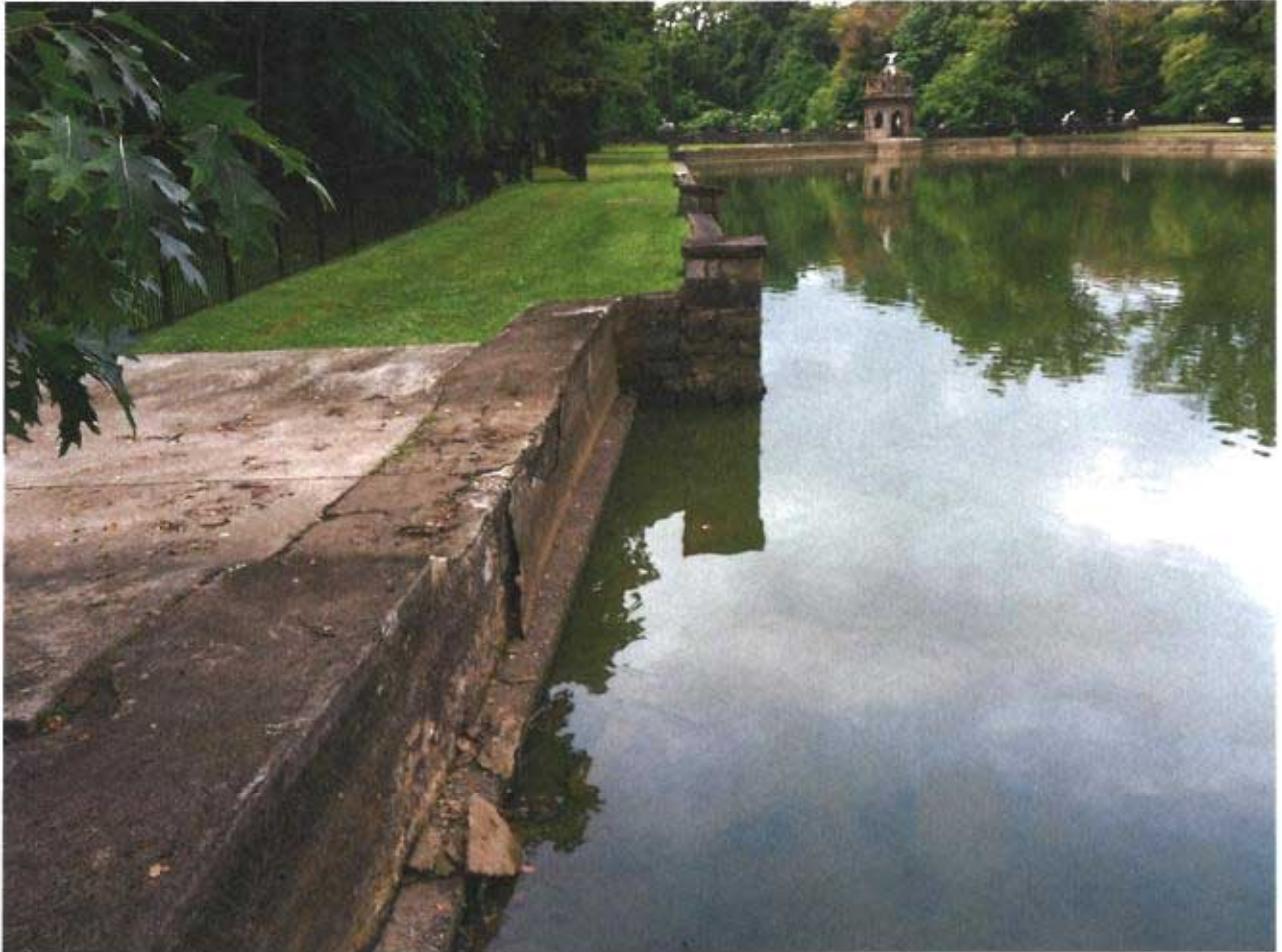
Loch Linden spillway (facing west):
