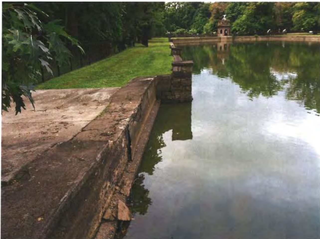
Loch Linden spillway (facing west):
