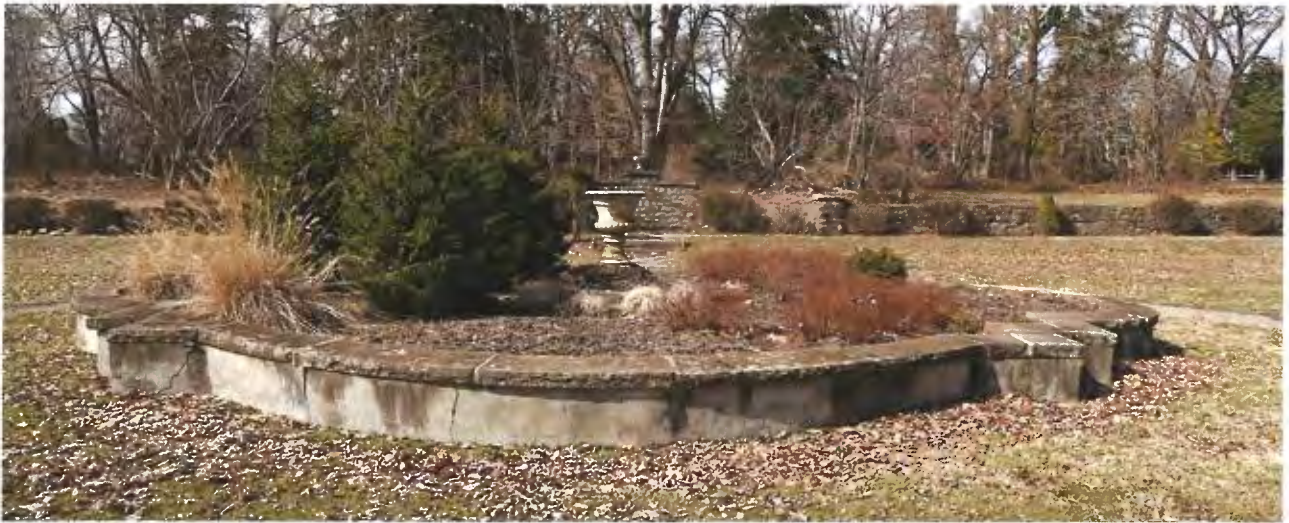
Sunken Garden Walls Top: Facing east Bottom: Facing west
