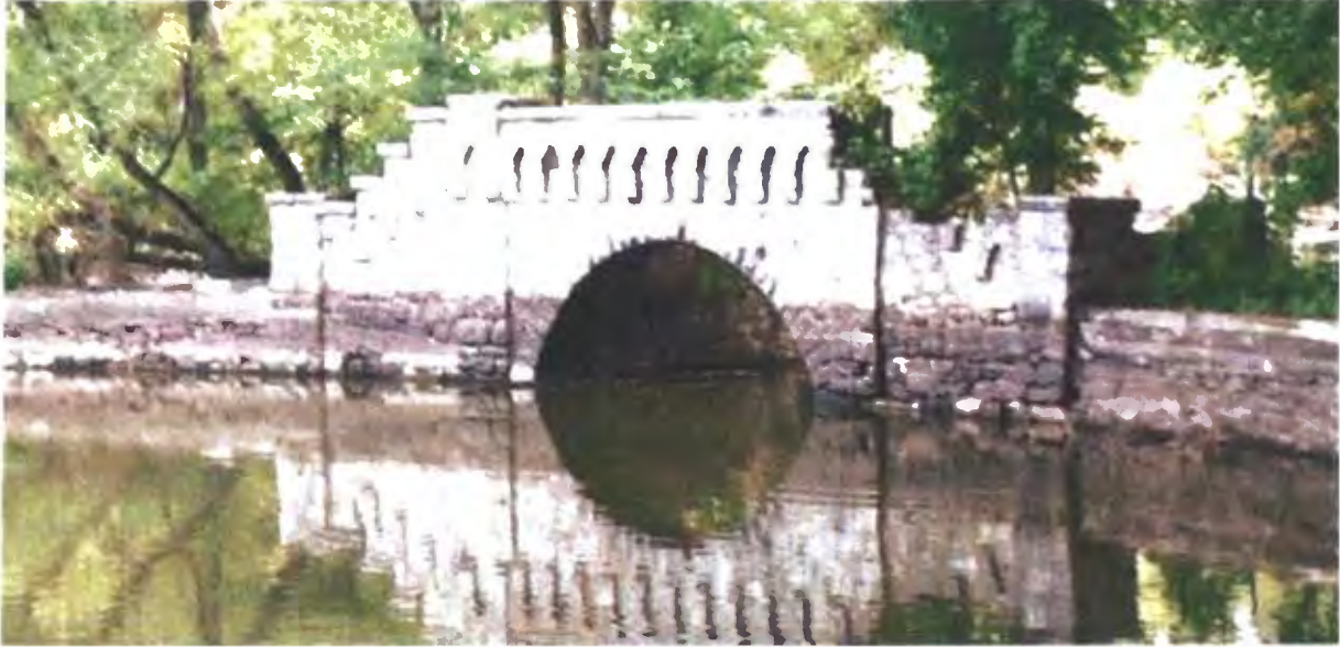
Loch Linden Arch: Facing northeast (top) and northwest (right)
