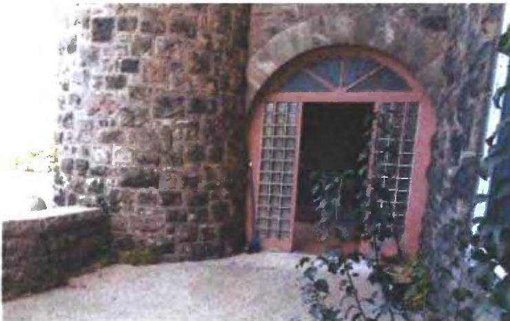
West Elevation Details: An arched doorway connects porch to a raised, open patio to its north. The doorway features a glazed fanlight transom and glass block sidelights in wood frames, but no central leaf. The patio features a concrete floor and a low stone-capped perimeter wall.
