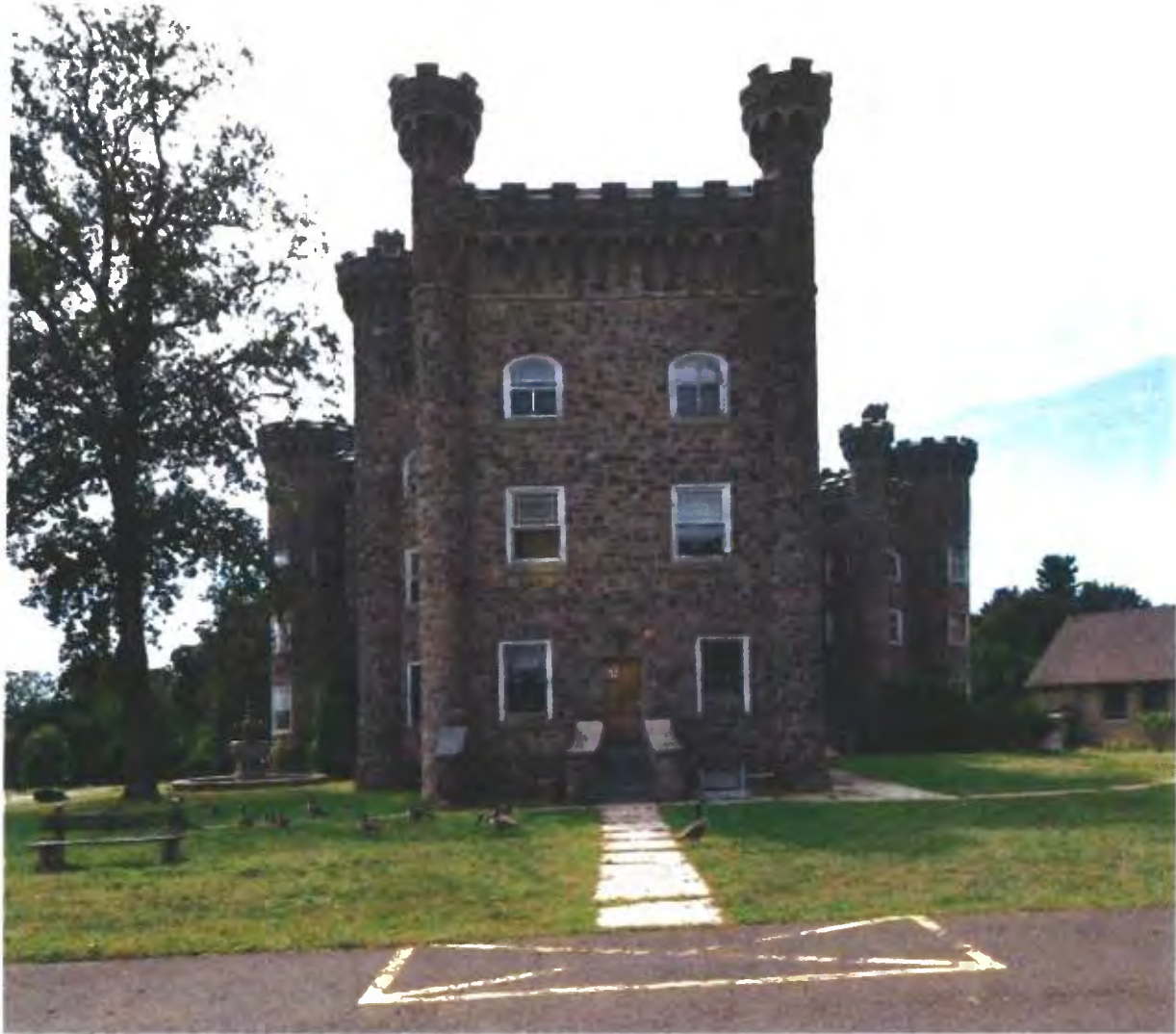
East Elevation: The building's three-story rear ell faces east with a two-bay elevation bracketed by slender blind corner turrets crowned by ornamental battlements. A single-leaf wood door is centered on the ground floor, accessed by a narrow stone stoop framed by thick sidewalls.
