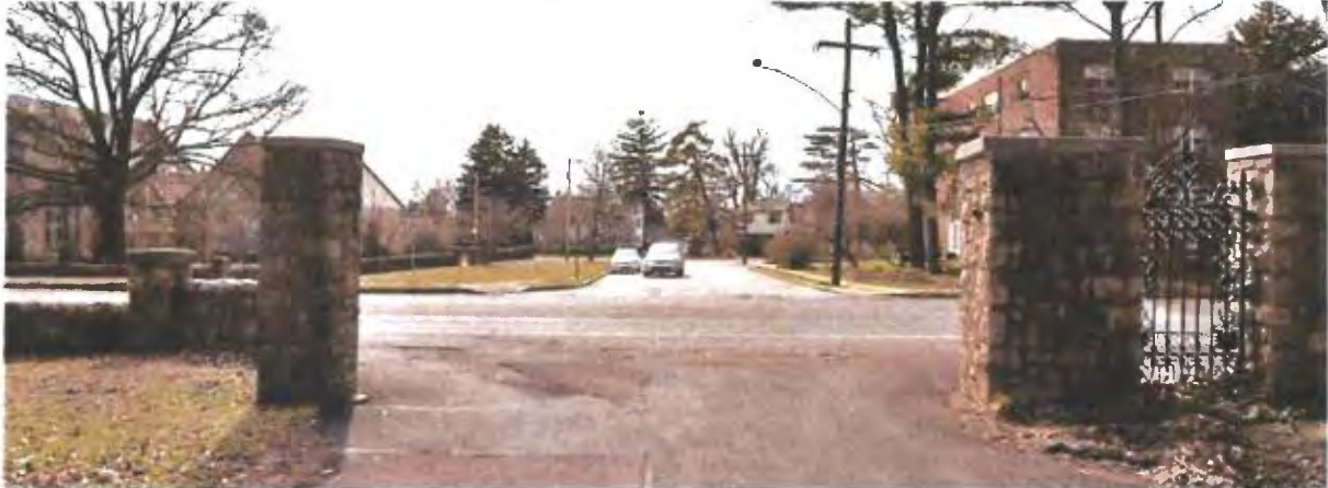
Bethlehem Gate Top: Facing west Right: Gate detail
