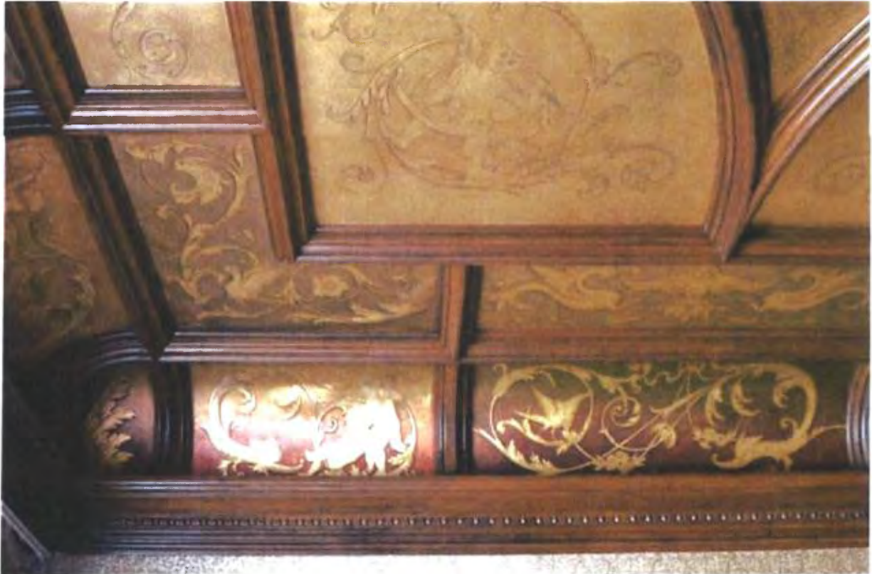
First floor library details: (Top) Painted ceiling panel detail. (Right) Book case detail
