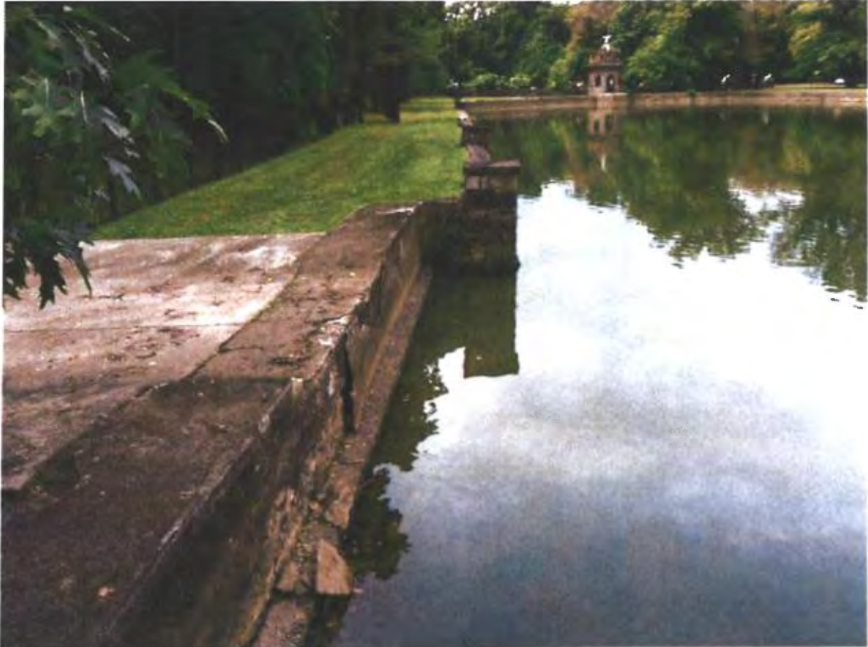
Loch Linden spillway (facing west):
